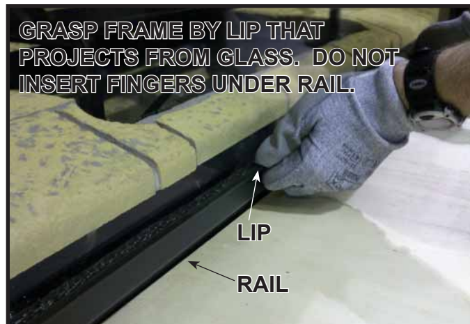
Figure 11.6. Installing Glass
