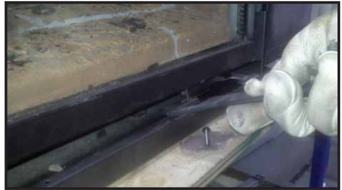
Figure 11.2. Glass Clip Tool Location
