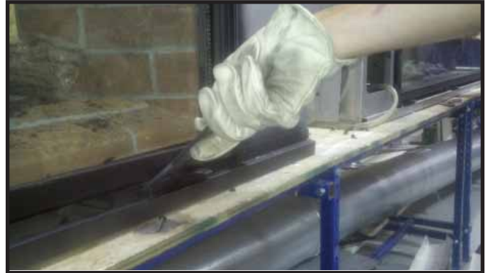
Figure 11.3. Inserting Glass Clip Tool
