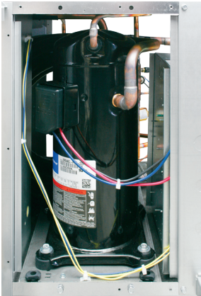
Double grommet compressor isolation
