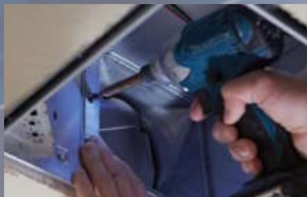
For room-side installation, pull the duct through the opening, attach the duct to the connector, push the connector into place and fasten to the housing with only one screw.
