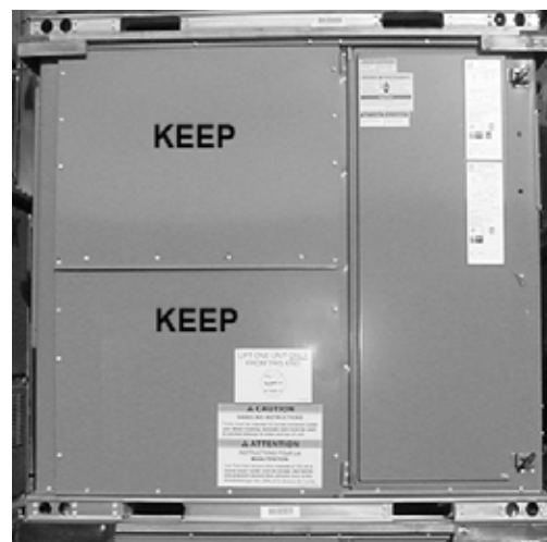
Figure 20: Save Side Panels For Economizer Hood Tops
