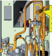
This is the position of the 4-way valve. Do not touch it directly with your hands. There is hot refrigerant at the discharge pipe, so be careful not to be scalded.
