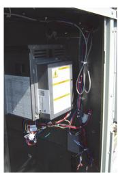
Figure 7. Factory installed VFD assembly
